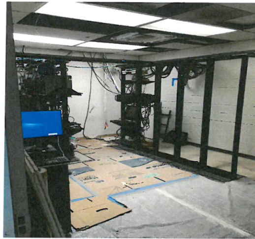
IT Room under Construction
