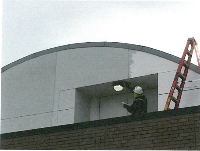
Roof Stucco Repairs
